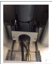
Step 10: Install four safety plates, four electromagnets and the electromagnet covers. Connect the wire to electromagnets.
